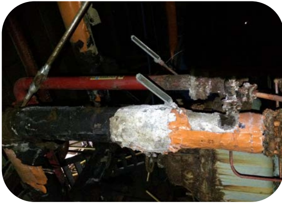
Pipe Insulation & Muddied Fittings (Mech Room)
