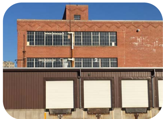
West Elevation Windows (Caulk & Glazing)
