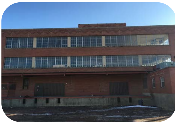
North Elevation Windows (Caulk & Glazing)
