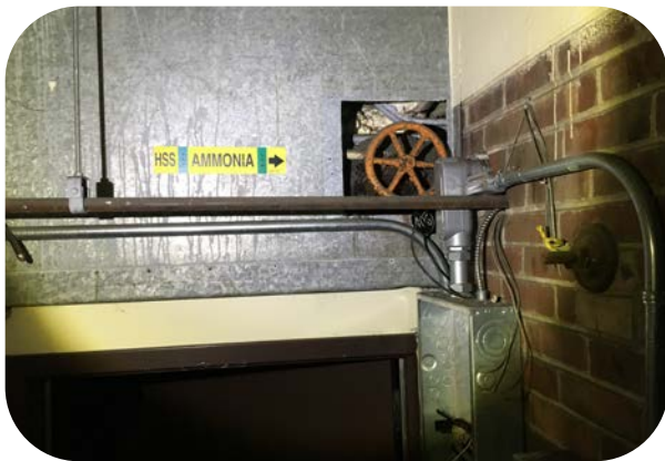
Pipe Mastic (1st Floor Stairwell)
